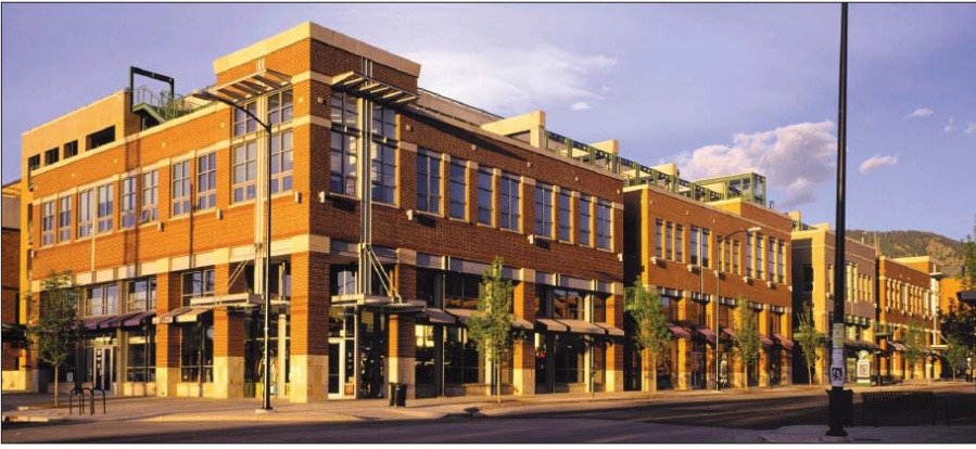
Above: The strategic and efficient distribution of shared parking leverages what is often a burden into a resource that can actually produce real estate, as shown above in the "liner" building concealing a public, shared garage.
